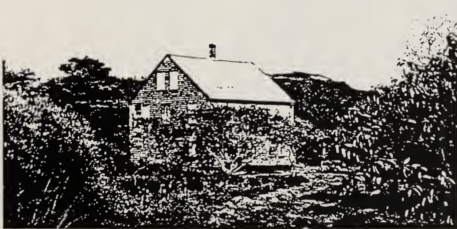
Bog House - Tract #17-2706 Bldg #T-17-23
